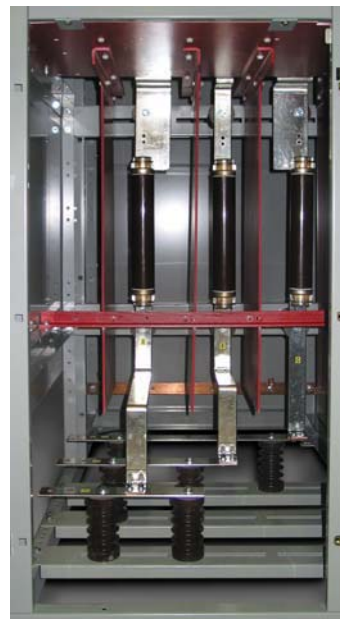
Main bus design with fuses
